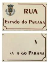
Figure 4. Castelo Branco Toponym PVC signage with information disposed on trimmed vinyl applied on top.
